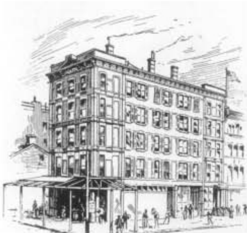
THE HOUSE AT 302 WEST 47TH STREET, NEW YORK
